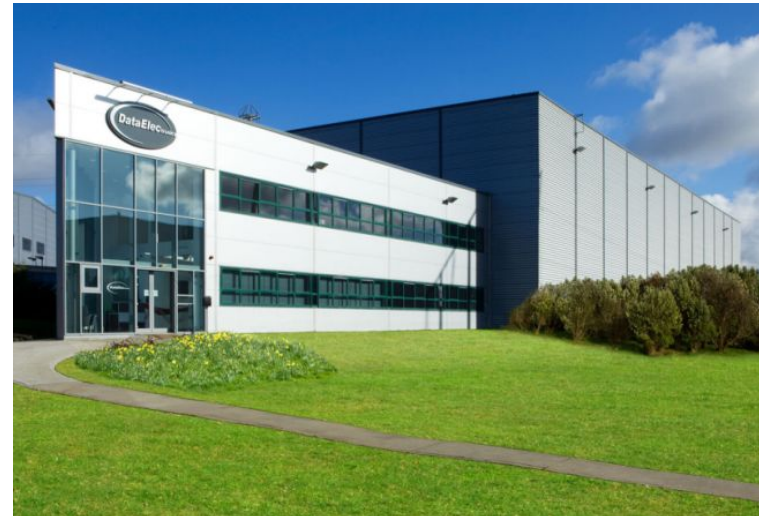
Northwest Business Park Data Centre
